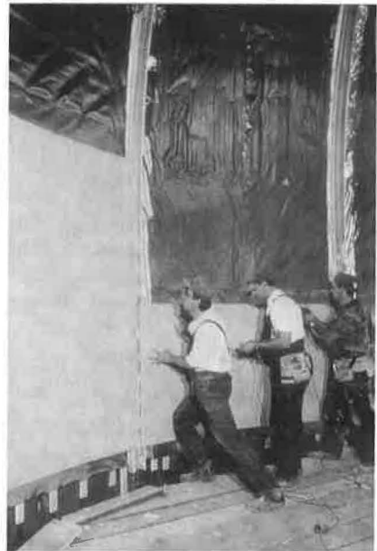
Figure 4: Attachment of gypsum plasterboard to the substructure
