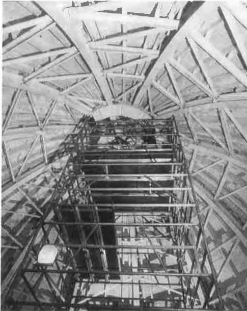
Figure 3: Load-bearing substructure of the tower cupola
