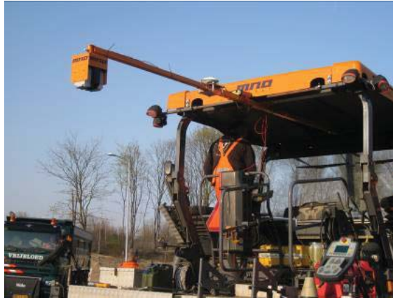
Figure 2: Linescanner mounted behind a paver
