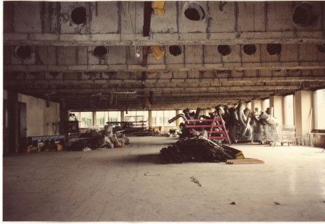
Figure 5. Office floor during construction. (Mitsui Fudosan archive)
