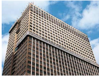
Figure 14. Exterior wall painting with full-circumference scaffolding. (Mitsui Fudosan, 1999-2015)
