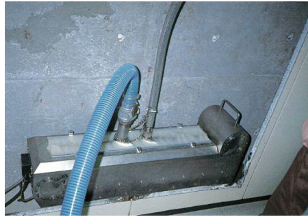
Figure 12. Opening work by rotary water jet method. (Mitsui Fudosan, 1989-1994)
