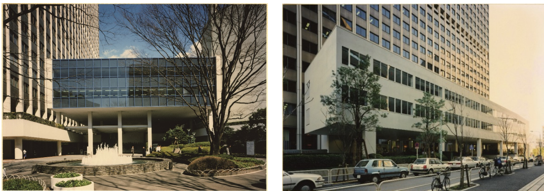
Figure 10. East(left) and west (right) provisional transfer office buildings. (Mitsui Fudosan archive)
