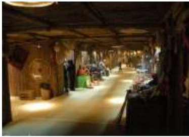
Figure 23: Roofing by Palm Rachis in in Qattara Heritage village in UAE (Piesik,2012)
