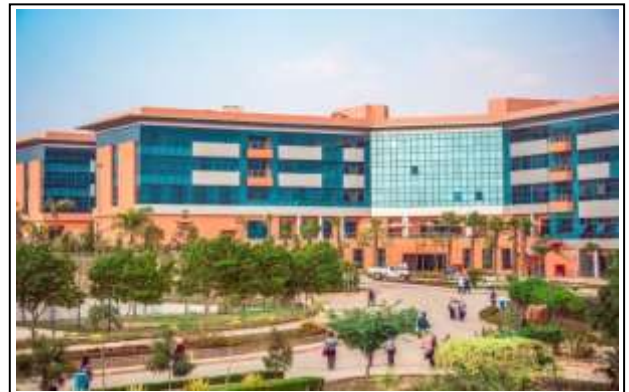
Figure (8): D-Building in the German University in Cairo (Author. 2016)
