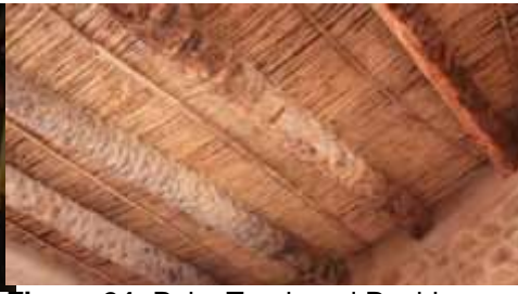
Figure 24: Palm Trunk and Rachis used for traditional roofing in Sinai.(Ibrahim, 2010)
