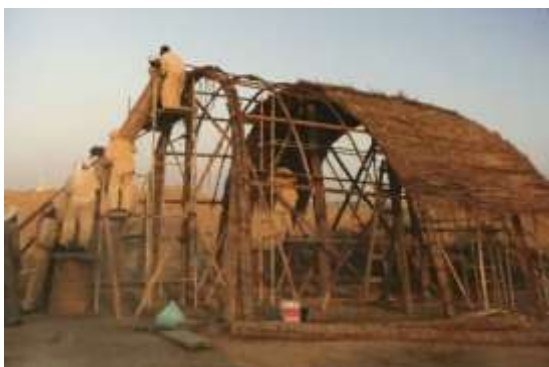
Figure 32: The Vault during Construction (Piesik,2012)
