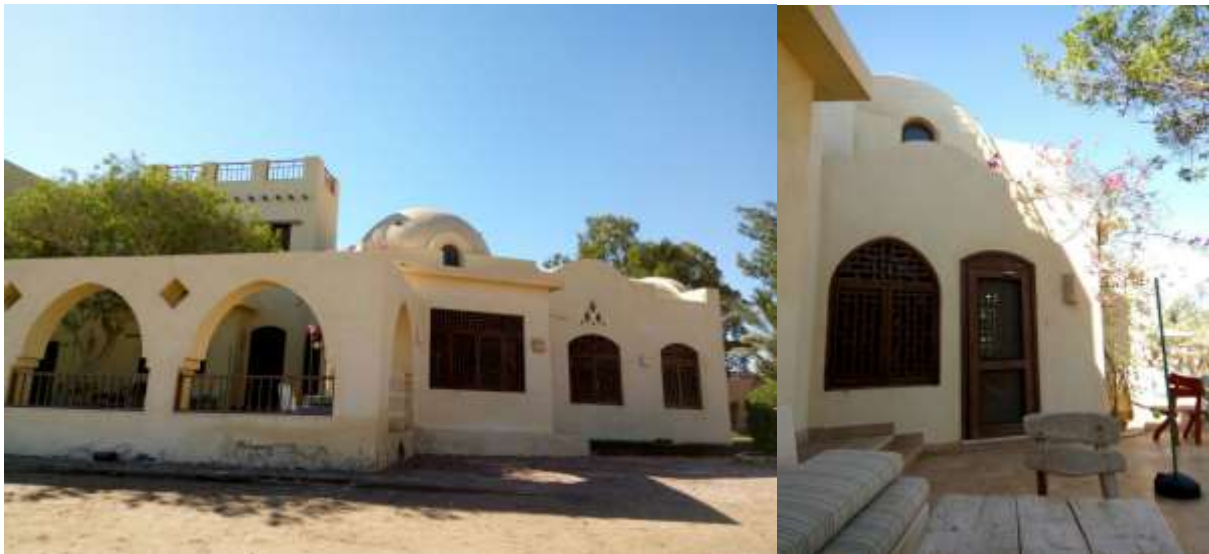
Figure 62: Villa in El Gouna, based on bearing walls Photo: Hend El-Dahan
