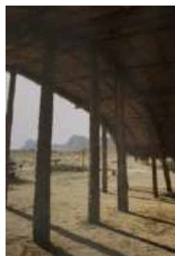
Figure 33 : Interior Columns (Piesik, 2012)
