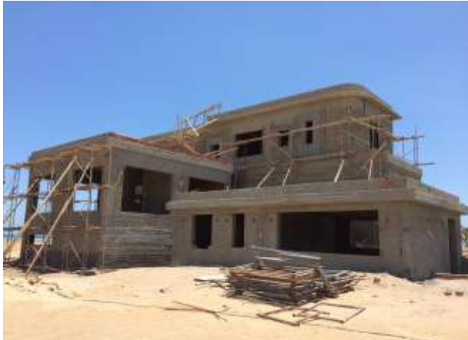
Figure 60: Construction site of a single family house in El Gouna
