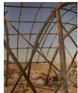
Figure 34: Rope based Connections.(Piesik,2012)
