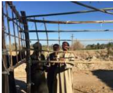
Figure 30: Adding vertical and horizontal bracings (Author)
