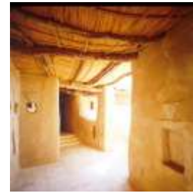
Figure 25: Roofing by Palm Rachis Adreere Amellal Eco-Lodge( Alamuddin, 2001)
