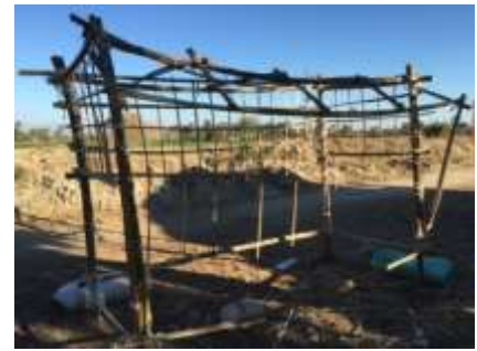
Figure 31 : The Shade after Completion (Author)
