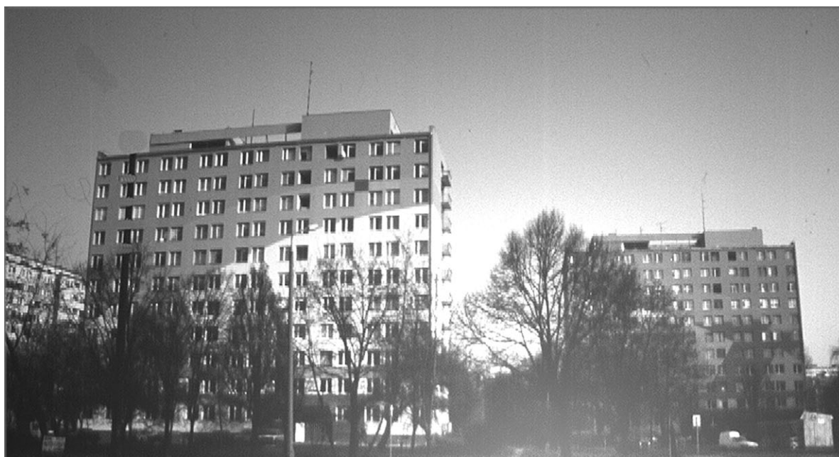
Fig. 4 The complex thermal renovation made in 2001 of buildings of co-operative housing estate "Anna" erected in 70s with modernized fire protection systems and repaired roofs (photo W. Szarejko)
