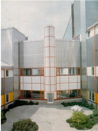
Figure 4: High-tech cladding has a higher capital cost value and might prove difficult to maintain.
