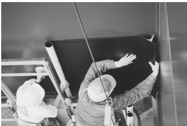
Picture2. The renewal construction work on a temporary scaffolding
