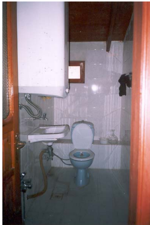
Figure 7. Interior view of the toilet in the office buildings in Buca.
