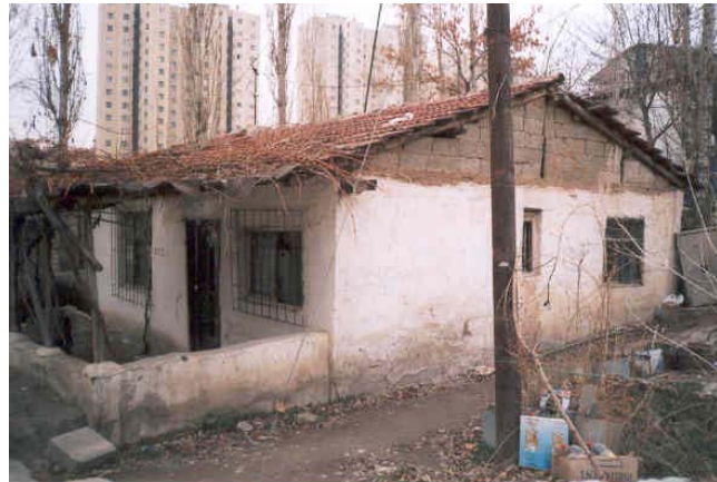
Figure 1. A squatter house in Ankara, built with salvaged material, mismatched windows and iron grills.
