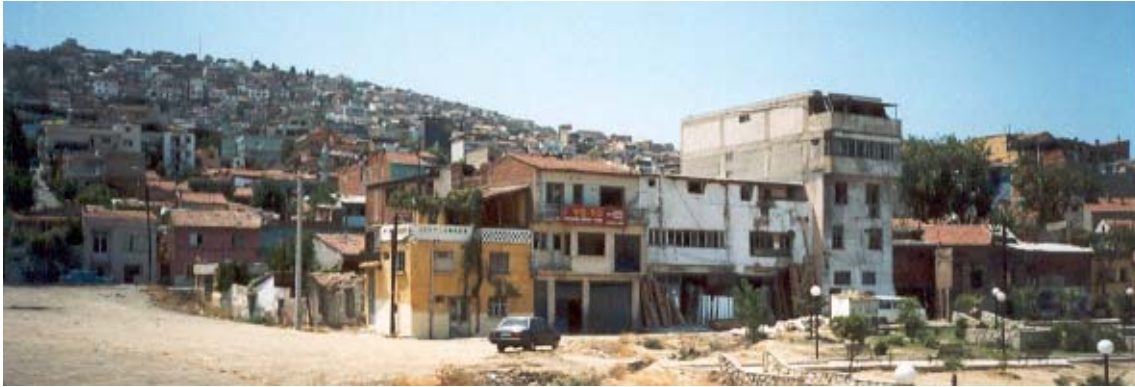
Figure 8. Low cost buildings showing evidence of incremental construction, with squatter housing in the background, in Izmir.
