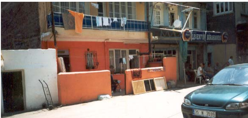
Figure 9. Low-cost buildings in Izmir, built with used building components.
