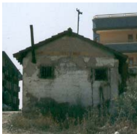
Figure 2. A squatter house in Ankara, built with salvaged concrete blocks that still have bits of old plaster and paint sticking on them.
