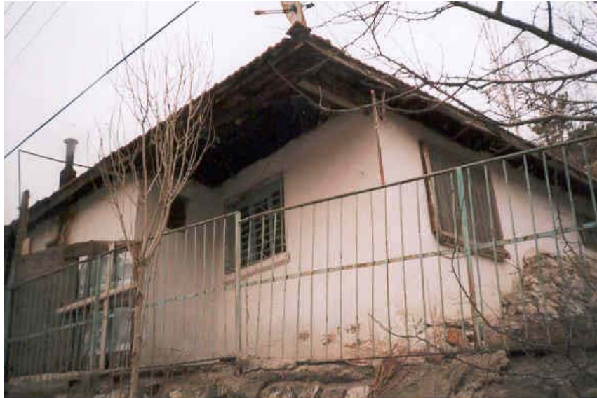
Figure 3. A squatter house in Ankara: the iron-grills are rotated to fit the windows.
