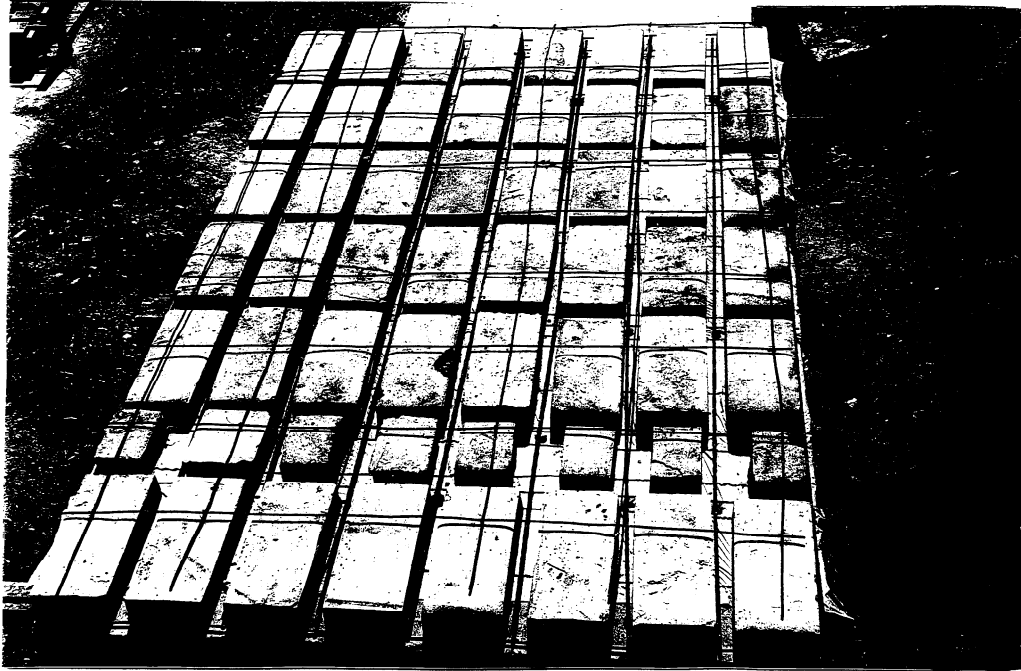
Fig. 2 RC filler slab under construction
