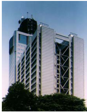
Figure 2 After the retrofit
