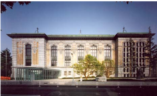
Figure 10 Main entrance elevation after the retrofit
