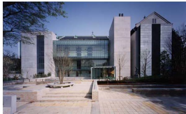
Figure 11 Courtyard elevation after the retrofit
