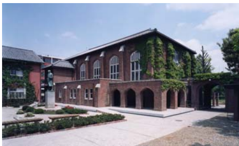
Figure 7 Exterior after the retrofit
