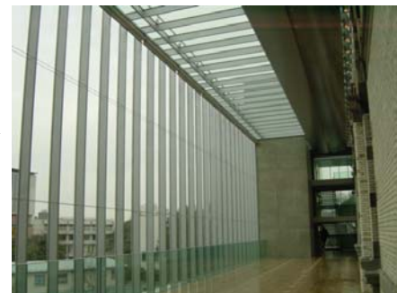
Figure 14 Steel plate column-mullion
