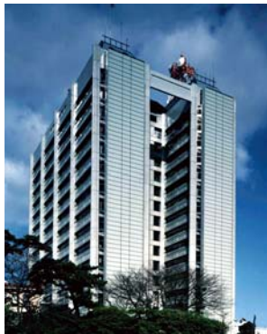
Figure 1 Before the retrofit
