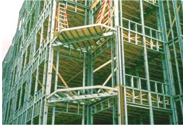
Figure 5 Multi-story from CFS sections
