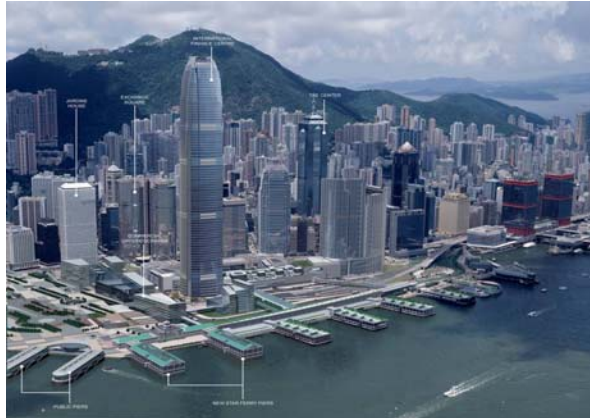
Photo 1: Two International Finance Centre
