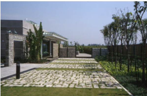
Figure 1 Southern entrance of Phase 1 building with granite from Police Headquarter's wall as paving; Gabion wall with oyster shells from Lau Fan Shan oyster farm
