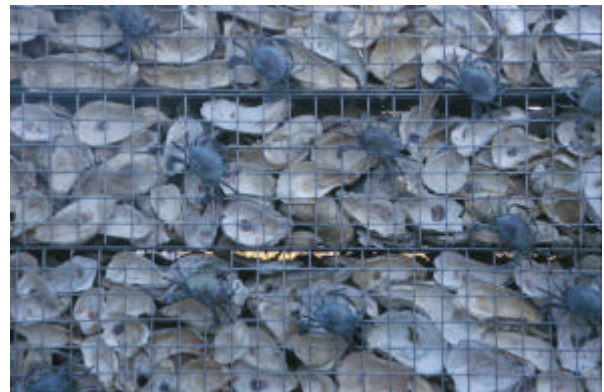
Figure 1 Southern entrance of Phase 1 building with granite from Police Headquarter's wall as paving; Gabion wall with oyster shells from Lau Fan Shan oyster farm
