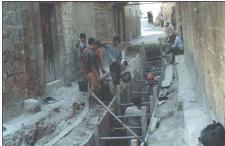
Photo 2 Renovation of infrastructure in the Old City alleys.
