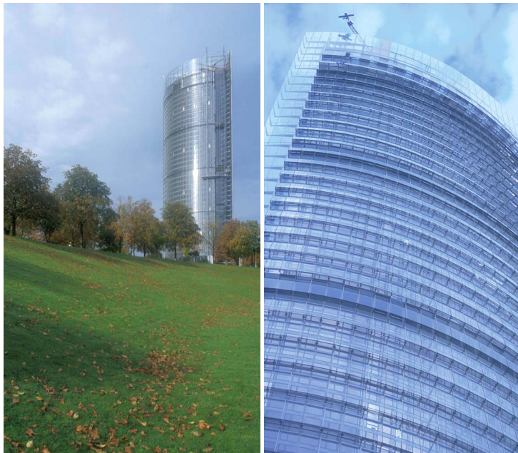
Figure 1 Views of the building. Source: Anja Thierfelder, 2003.
