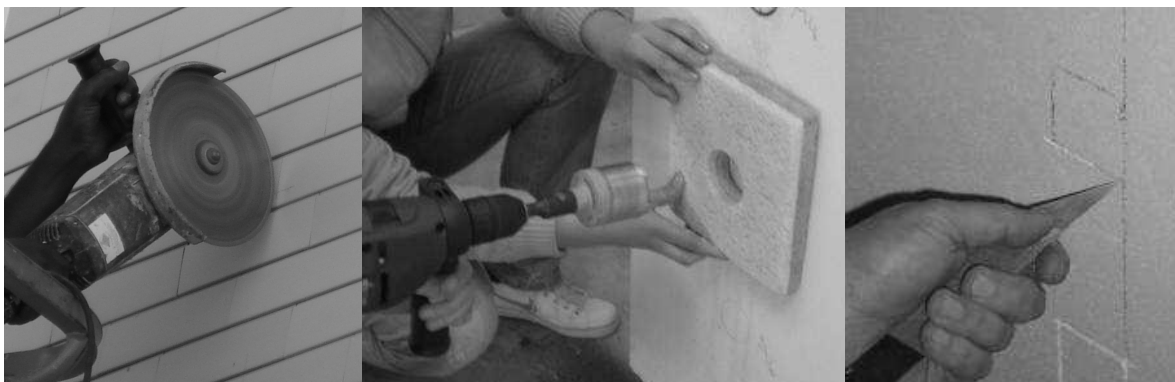
Figure 2. Pre-cut a) ceramic tiles, b) rendering, c) ETICS
