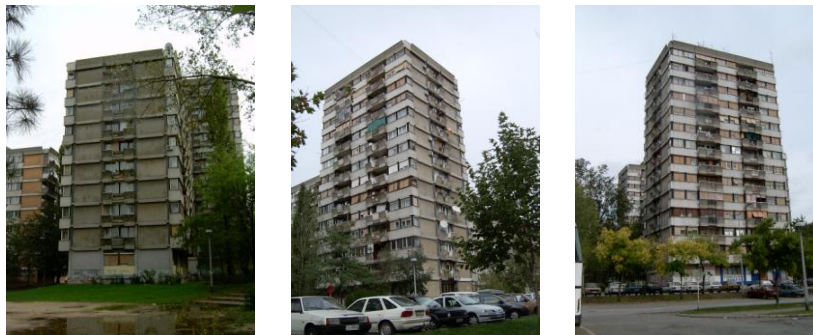
Figure 3. Residential towers S-3 (P+9), S-4 and S-6 (P+14) Liman III-1 block;
