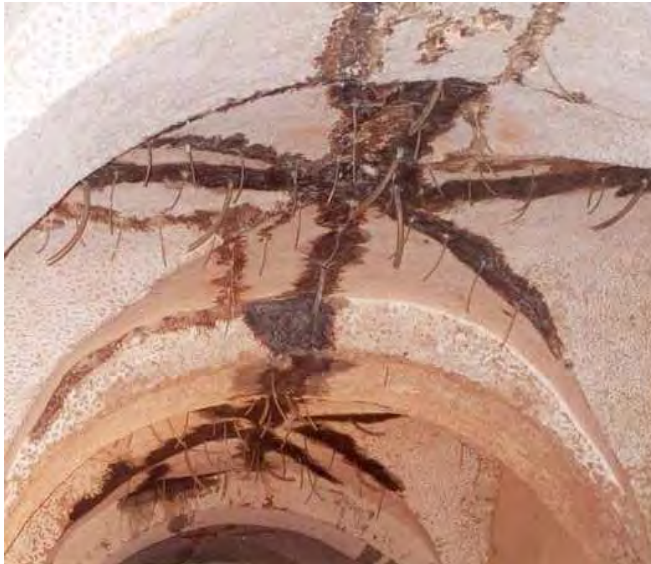
Figure 26: Injections of epoxy resins in a masonry vault (21)
