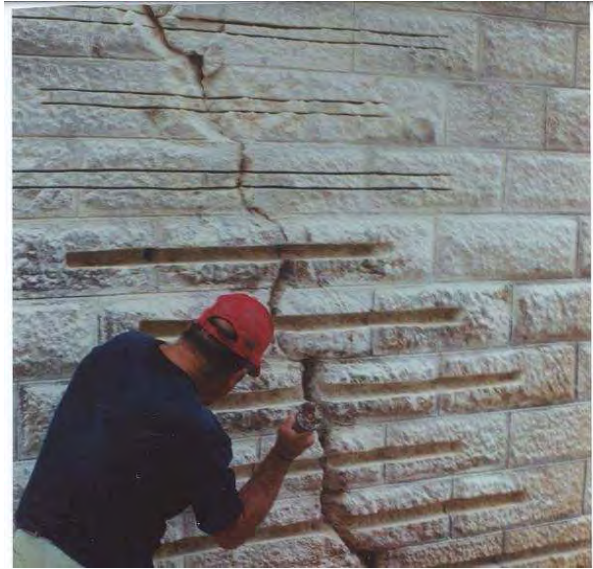
b) With clamps in cracks (21)
