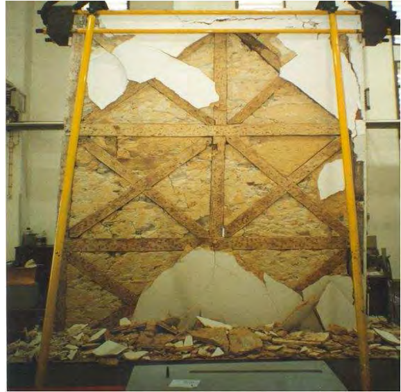
b) The wall after tested
