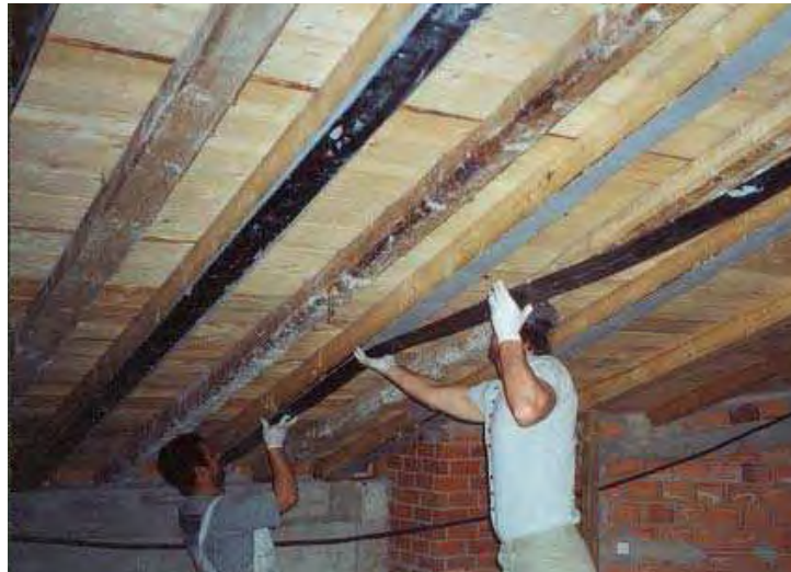
Figure 33: Strengthening of timber floor with composites (20)
