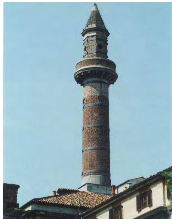
Figure 32: Tying of masonry tower with steel strips (21)
