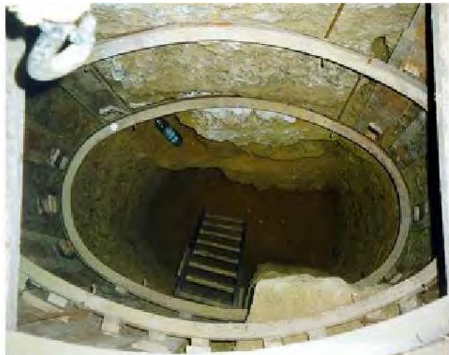
Figure 16: Shaft for the geotechnical recognition of building foundations (21)
