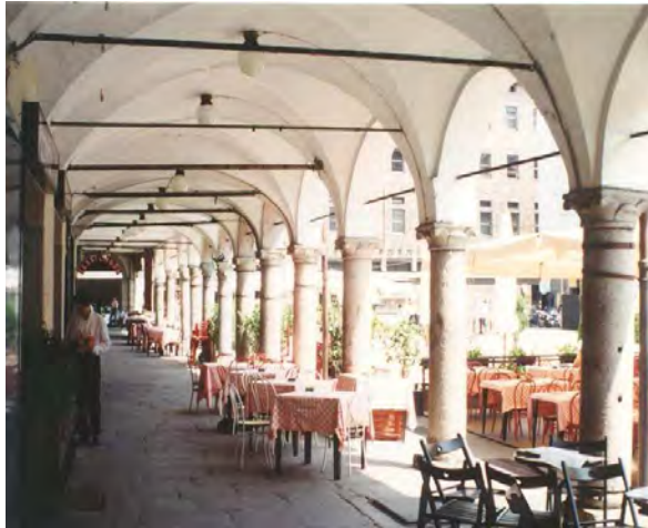
Figure 30 Tying of masonry vaults with tie-rods in steel (21)
