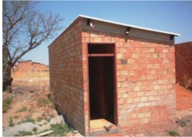
Fig 8. A house unit which is poor in sound and thermal insulation in Hlalanikuhle Housing, Bulawayo. Source: Author, 2006.
