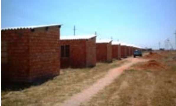
Fig 3. Dust access road of Hlalanikuhle housing, Bulawayo. Source: Author, 2006.
