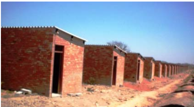
Fig 5. Monotonous view of Hlalanikuhle Housing. Source: Author, 2006.
