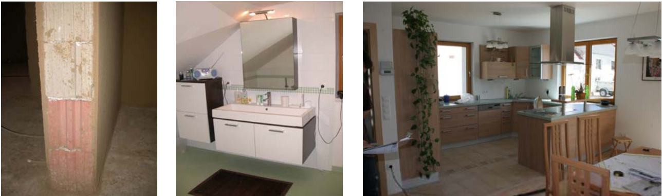
Figure 8: The loam plaster was executed with two layers and a reinforcement fleece in the first layer to ensure a good adhesion on fired as well as unfired loam bricks. The sorption capacity of the loam has a positive influence on the humidity of the rooms.
