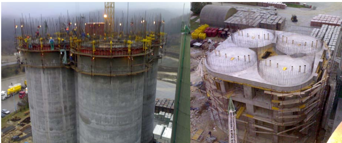
Figure 3: Chambers of the cement silo
