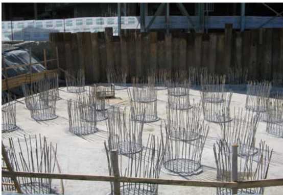
Figure 4: Reinforced concrete pilots
