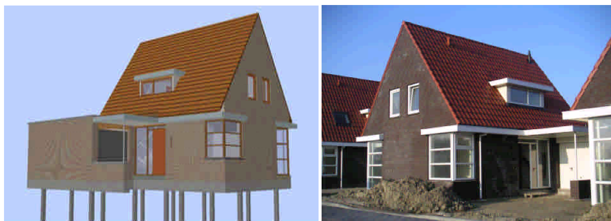
Figure 3: A 3D model and a picture of the pilot project of small-scale housing development in Zeeland, The Netherlands, with integrated design and BIM application
