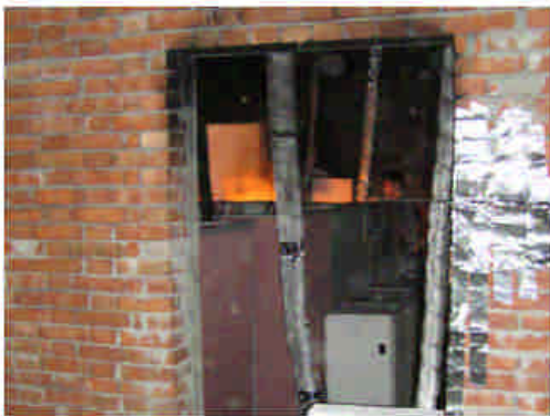
(a) View from the southern opening
