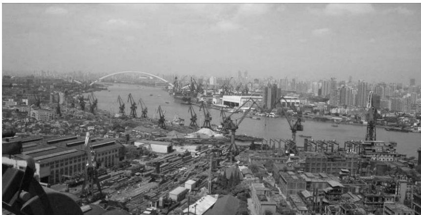
Figure 1: Pre-construction site view from Pudong (River East) overlooking Puxi (River West) with the vista of Lujiazui Financial and Trading Zone (as of May 2006)
