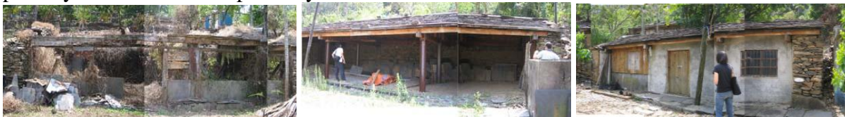
Figure 2: The process of refurbish slabstone houses
