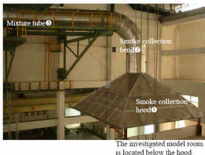
Fig. 1 : 10 MW fire test facility
