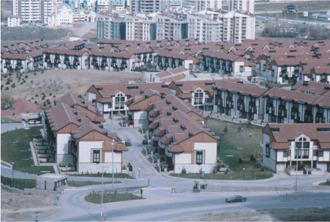
Figure 4. Batikent development: aerial view showing rows of modular housing
