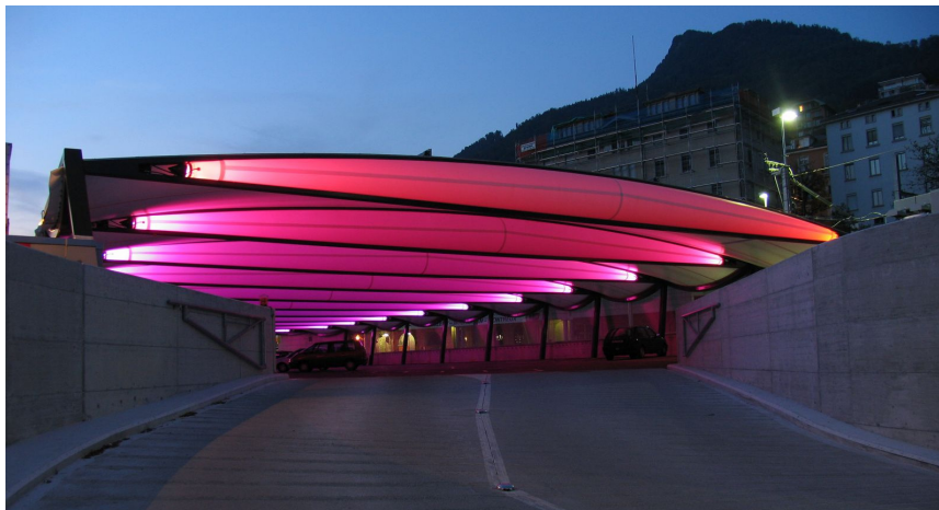
Figure 2. Tensairity roof structure in Montreux, Switzerland (Luscher Architectes SA).
