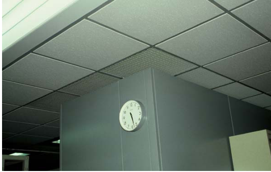
Figure 5. Ceiling panels and partitions
