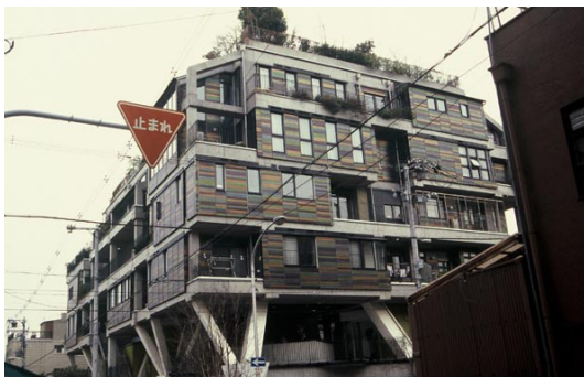
Figure 9. NEXT21 External Wall
