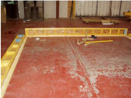
(b) Supports were fixed onto the timber frame using screws.
