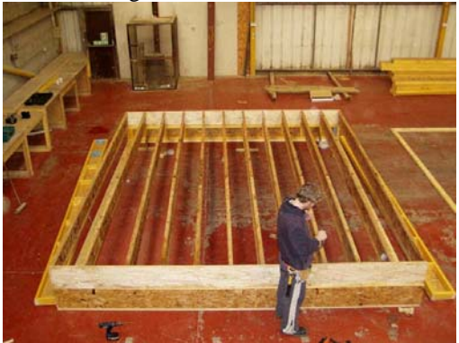
(c) The floor structure was constructed before placing decking boards.
