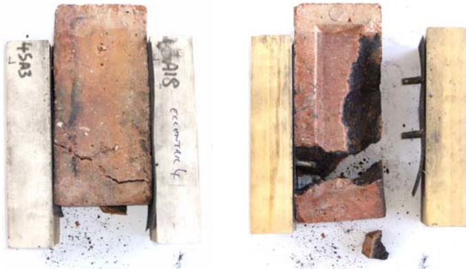
Figure 4.5 Propagation of cracks leading to the breaking up of brick substrate.
