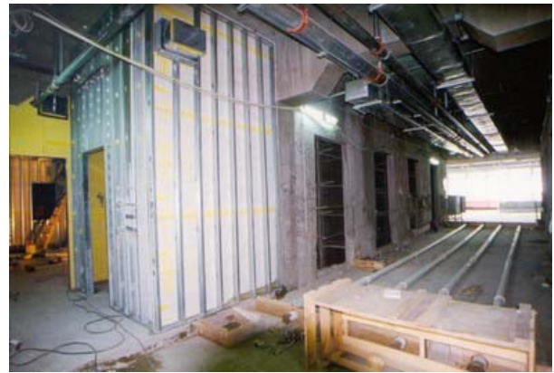
Photo 21 Dry wall installed as fire-resisting partitions
