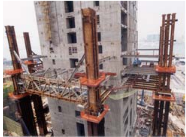
Photo 8 Mega-column erected from the raft and anchored on gusseted base
