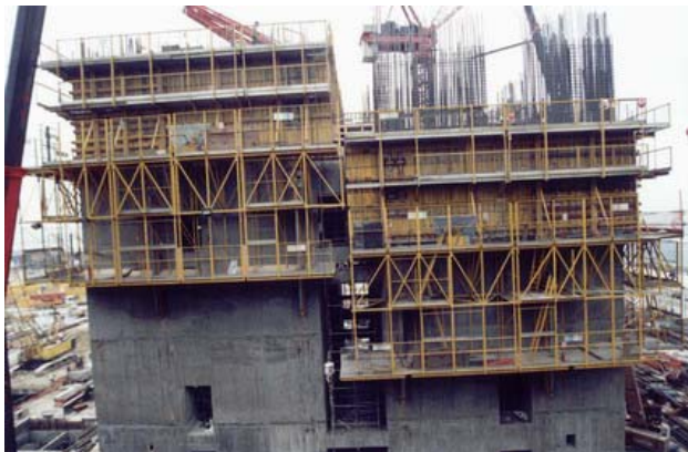
Photo 10 Climb form for constructing the core wall
