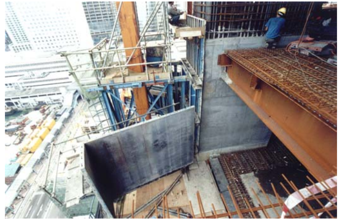
Photo 13 Detail of the form in its opened mode
