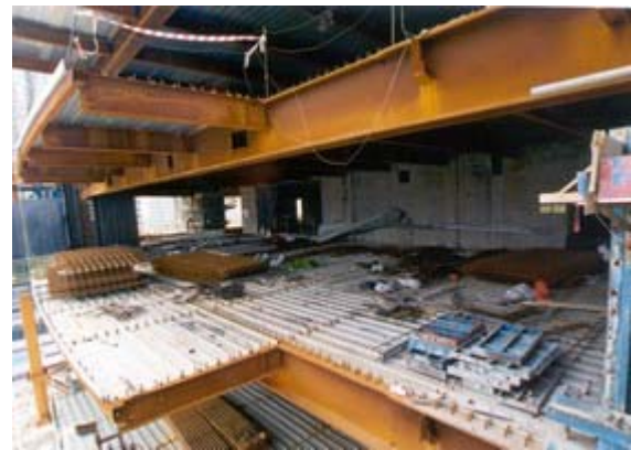
Photo 11 Girder beam spanning between two columns
