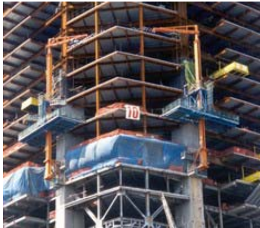
Photo 12 External mounted climb form for casting the mega-columns
