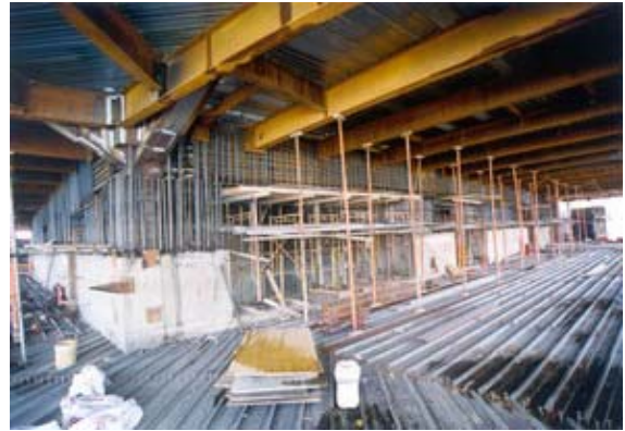
Photo 15 Encasing the anchor frame in a retro-approach
