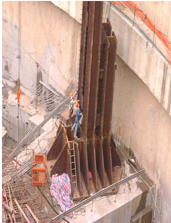
Photo 8 Mega-column erected from the raft and anchored on gusseted base
