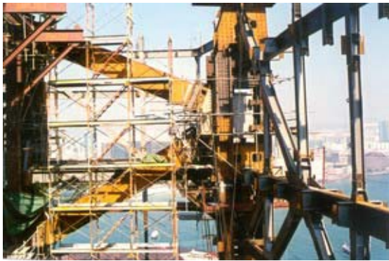
Photo 16 Jointing between outrigger and mega-column
