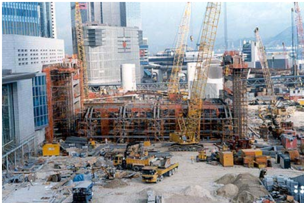
Photo 20 Construction of the link bridge
