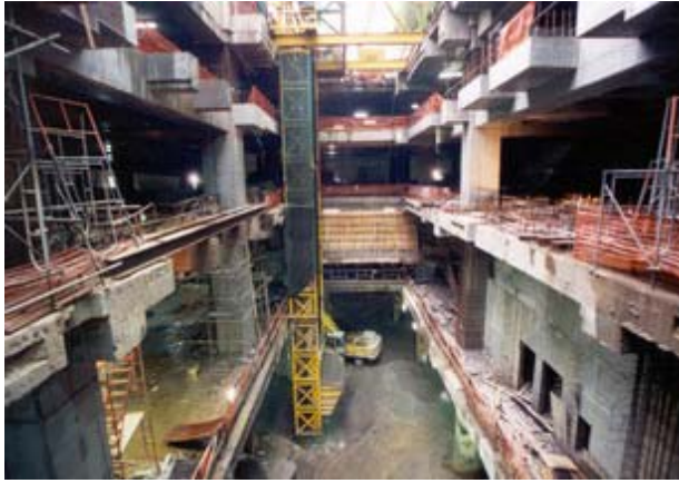
Photo 18 Temporary shaft for removing excavated spoil
