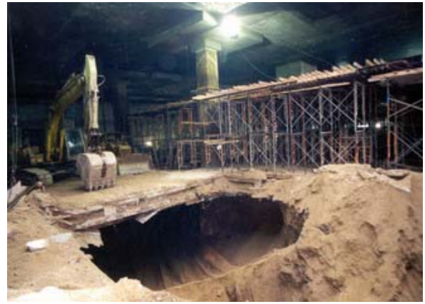
Photo 19 Typical double-bit construction arrangement
