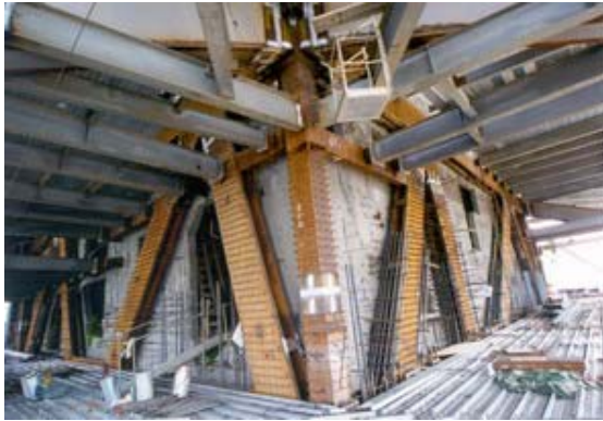
Photo 14 Inner frame as anchor for the outrigger system
