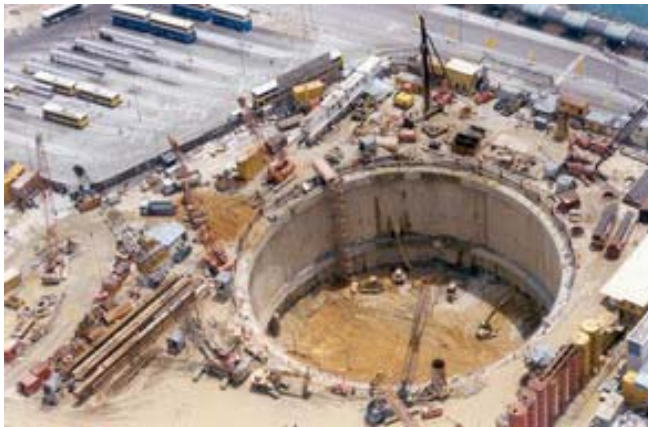
Photo 6 Cofferdam formed to house the 88-storey tower
