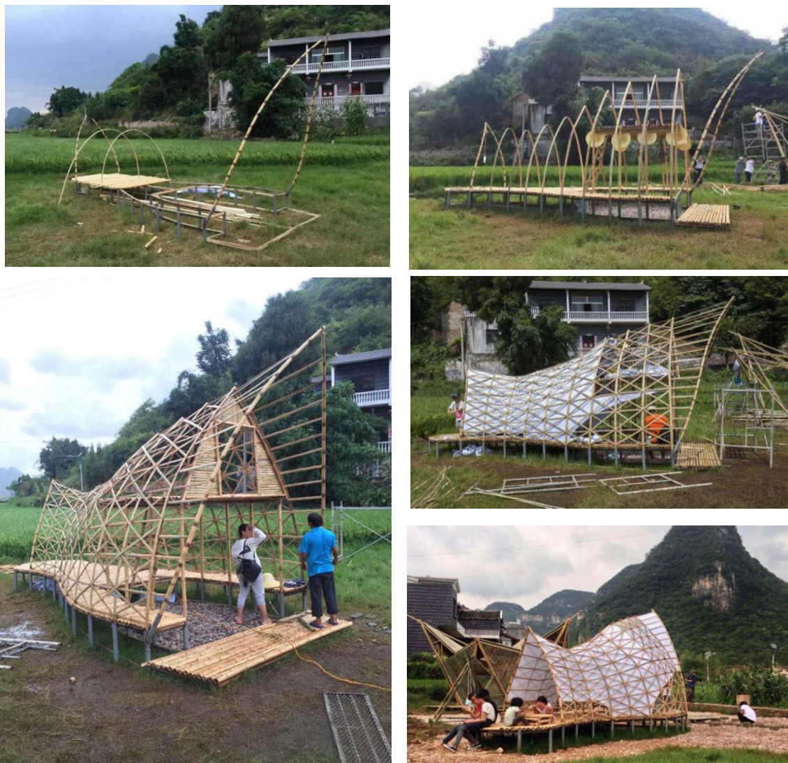
Figure 6:Field construction flow chart
