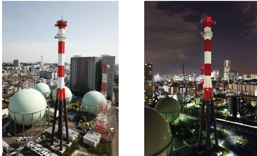
Figure 1: Overview of the new type of communication steel tower (daytime & nighttime)
