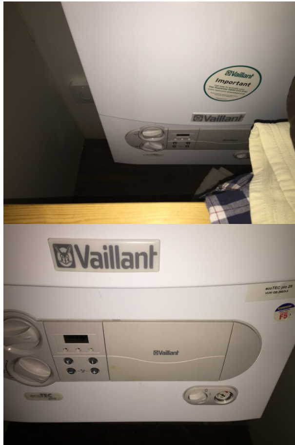
Fig 3. Above: photograph of boiler without model qualifier available, and below, boiler with model qualifier to right hand side (W-Y-P Gledhill, 2015)
