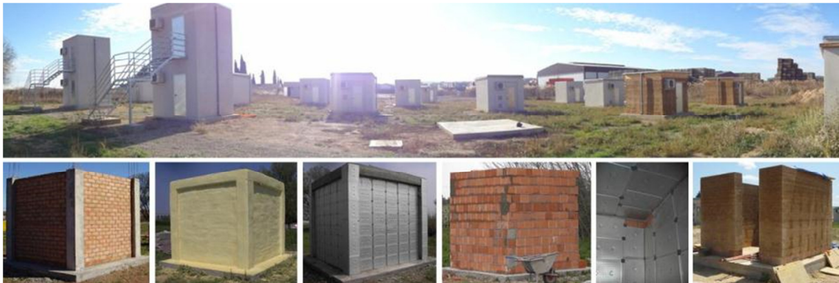
Figure 1. Experimental set-up located in Puigverd de Lleida (Spain). Up: general view. Down: cubicles during their construction, from left to right: BRICK, PU, PU-PCM, ALV, ALV-PCM, RAM.
