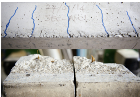
Figure 4. crack patterns of the concrete beam and rupture of bamboo composite reinforcements
