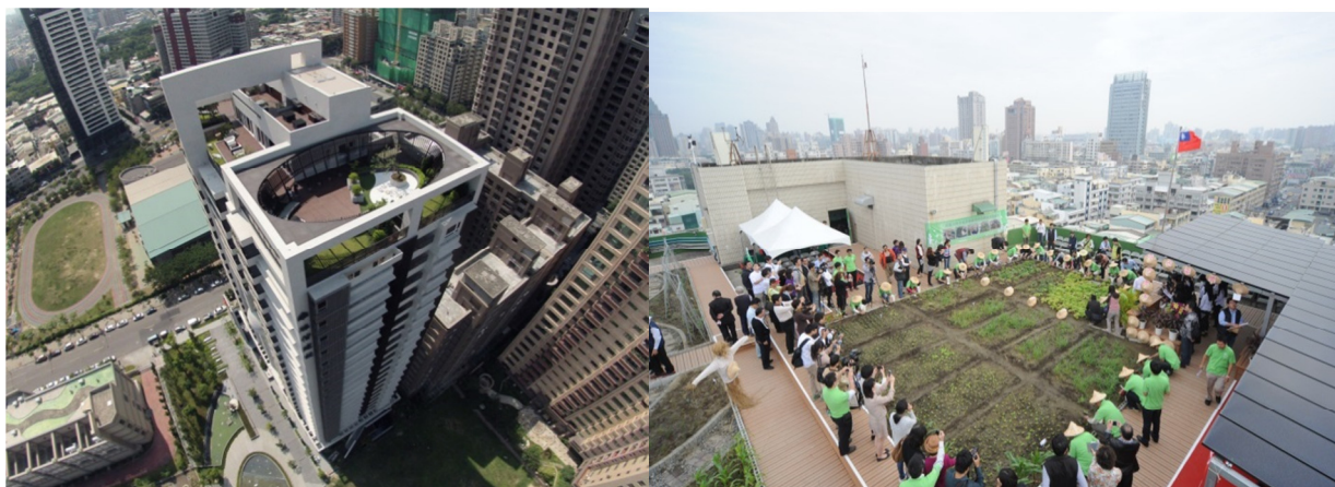
Figure 6. The pilot projects of green roof demonstration (left: Private high rise building, Right: the PV urban farming at the rooftop of Sanming district office)
