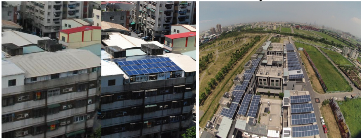
Before renovation (illegal) After renovation (legal) Figure 5. The pilot projects of PV roof demonstration
