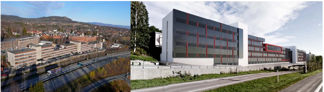
Figure 1. Solbraaveien 23 before and after refurbishment.
