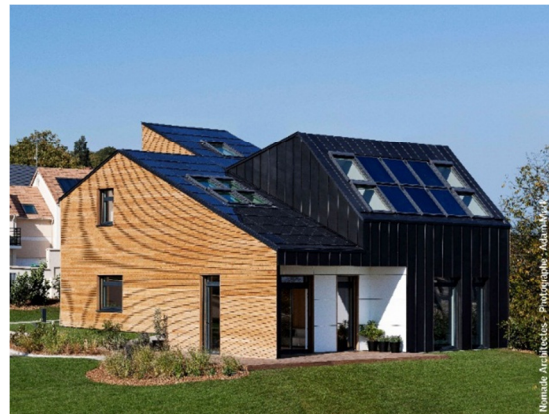
Figure 4: The nZEB Active House Maison Air et Lumière, located near Paris. © Adam Mørk 207
