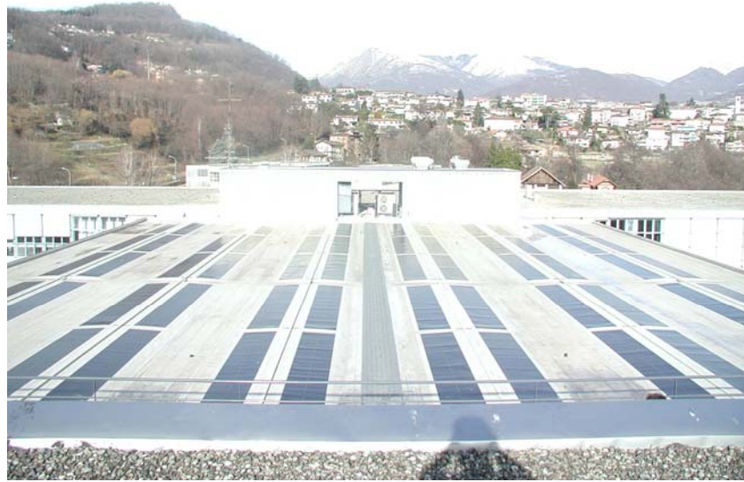
Figure 6 Flexible polyolefines (FPO) membranes flat roof laminated together with a 15.4 kWp a-Si triple-junction PV power plant.
