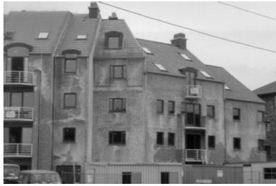
Figure 1. Example of efflorescence apparition at the end of work.
