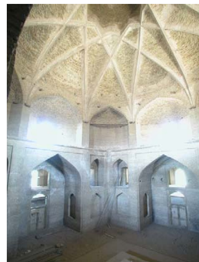
Figure 2. Inside the mausoleum with the cambered inner arch.
