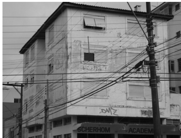
Figure 1. Facade of a construction with painting problems and detach of the plaster.
