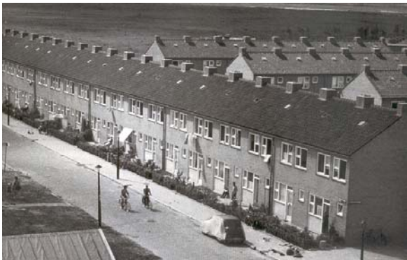
Fig. 1 Typical outdated row housing in the Netherlands (1953)
