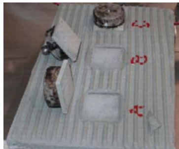
Figure 4 – Adhesive failure in the interface between the ceramic tile and the cementitious adhesive Sample PE0.
