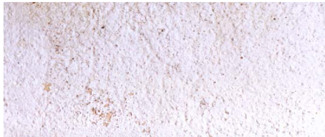
Figure 5. Aqueous polymeric disperse paints A2 after 85 cycles of complex effects (substrate – lime-cement mortar).
