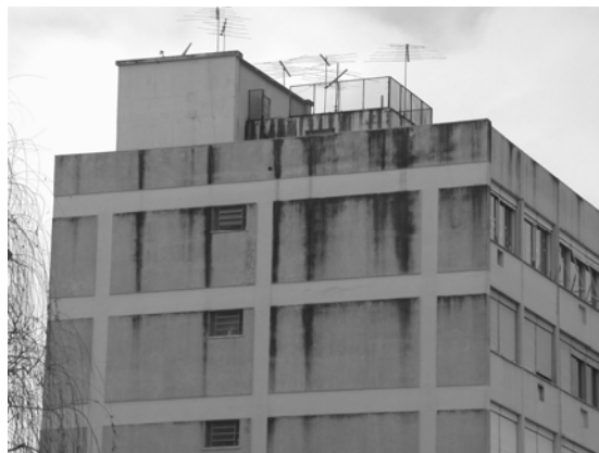
Figure 3 Moisture originated from the roof endangering the home of the last pavement.
