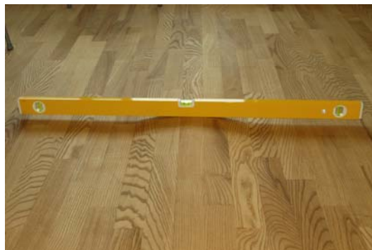
Figure 5. Swelling of wooden floor due to boards mounted without possibility for expansion in the humid season.
