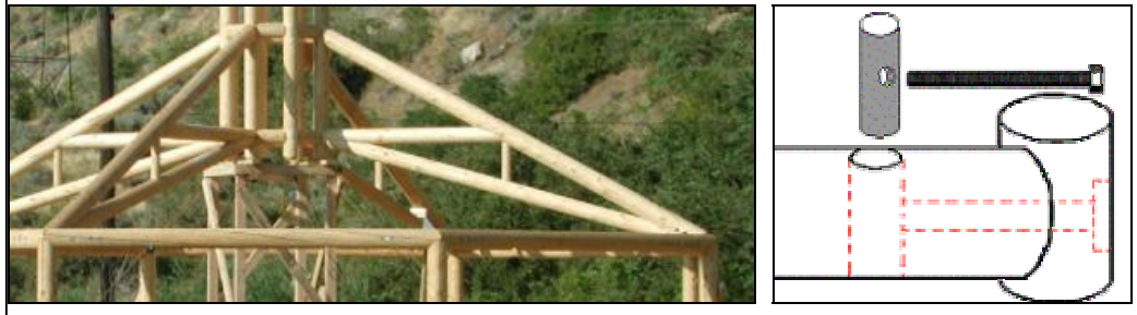
Fig.1 Round wood trusses (www.fpl.fs.fed.us)
