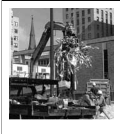
Figure 6 Recycling Metal from Bank One Building
