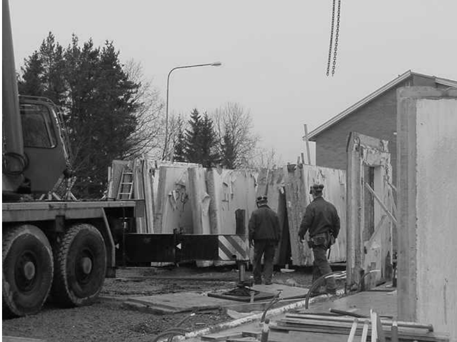
Figure 3. The concrete elements from the refurbishment project arrived at the building site in Linköping, Sweden.
