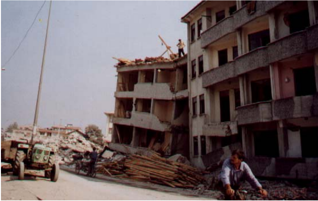
Figure 5: Recovery of building material from the severely damaged building in Figure 4; the structures beyond have been already been deconstructed and demolished [ij].
