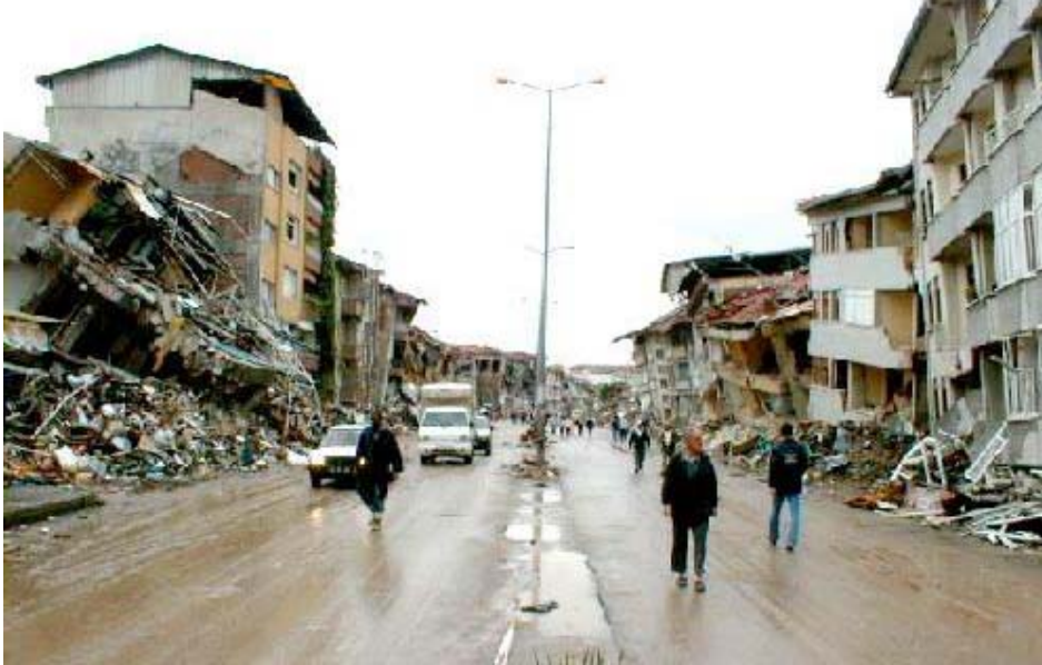
Figure 1: Extensive damage caused to the buildings located on one of the main roads in Adapazari, as a result of the devastating earthquake of 1999 in the Marmara region [ii].
