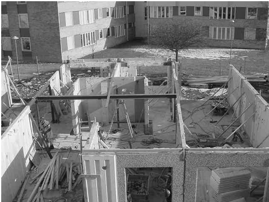
Figure 4. Frame construction in Nya Udden. Additional steel supports were used to further reinforce the building.
