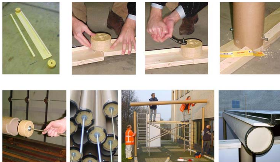
Figure 4. Pilot project - assembly sequences of intermediaries, columns, and beams
