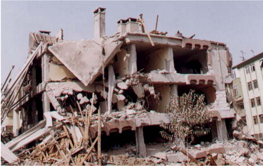
Figure 11: Dismantling the roof of the building in Figures 9 & 10 above [i].
