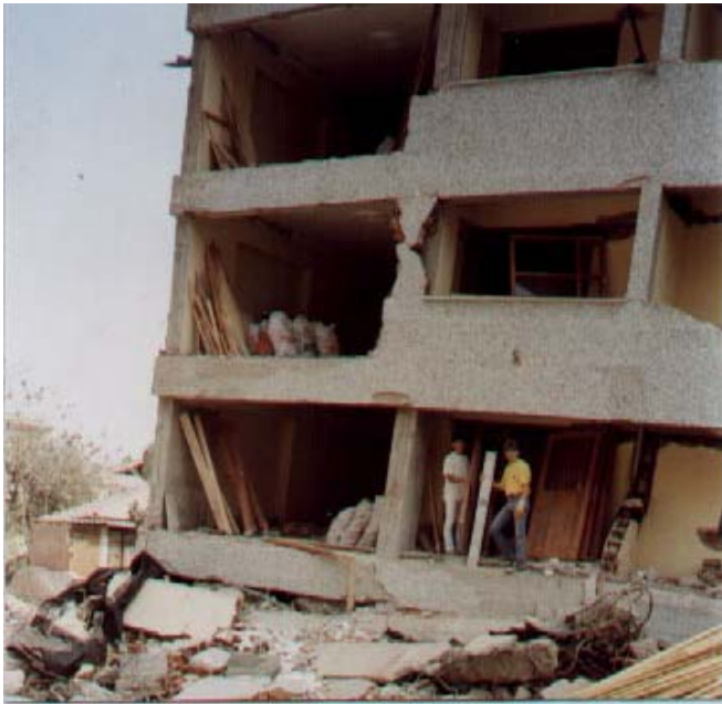
Figure 5: Recovery of building material from the severely damaged building in Figure 4; the structures beyond have been already been deconstructed and demolished [ij].
