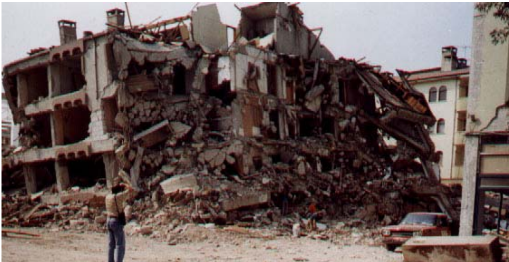
Figure 10: Removal of collapsed sections of the building shown in Figure 9 led to the collapse of an upstanding one at the rear, bringing down the penthouse with it [ij].
