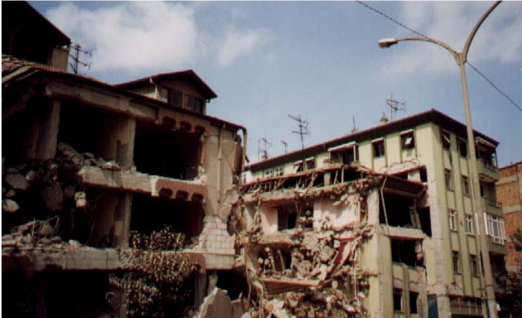
Figure 9: Partially-collapsed buildings with penthouse on the structure to the left [v].
