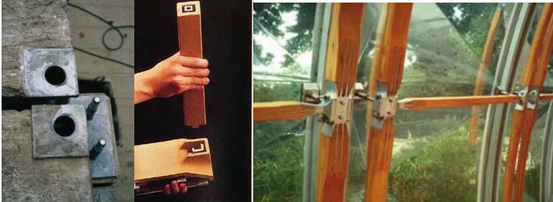
Figure 8: Steel as an intermediary between concrete floor components, brick components, and wooden structural elements.
