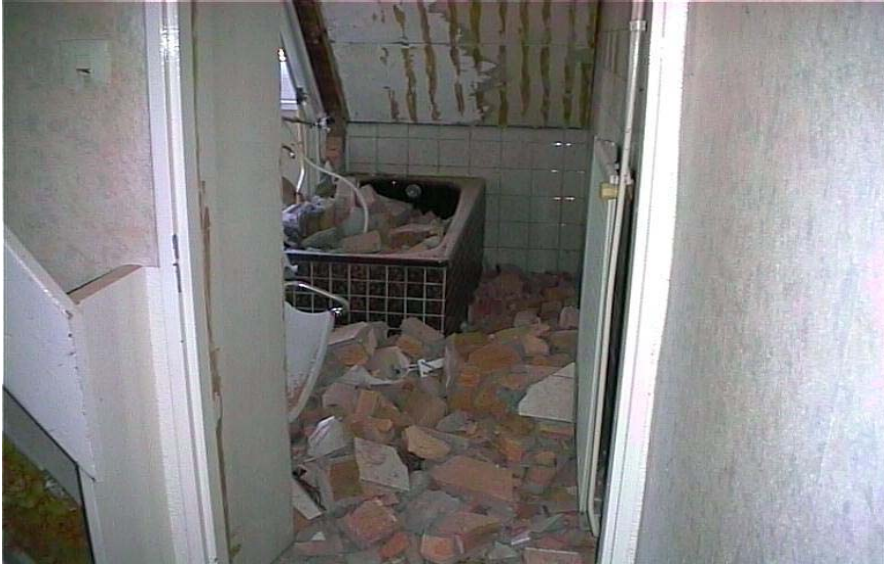
Figure 8 A bathroom with some demolished components, but... too many.
