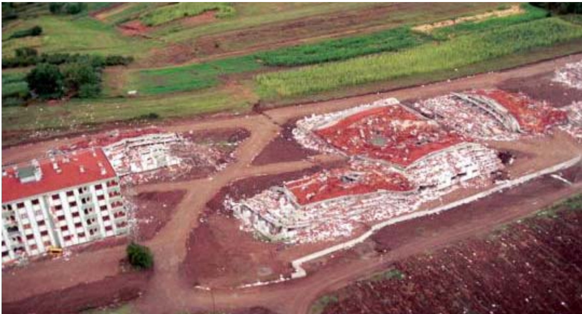
Figure 3: A moderately damaged building next to totally collapsed ones after the earthquake in the Marmara region [ii].
