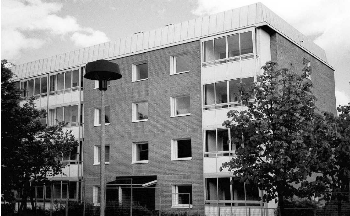
Figure 1. This is one of the apartment buildings in Finspång, Sweden that was torn down and functioned as a material source for a new building in Linköping, Sweden.
