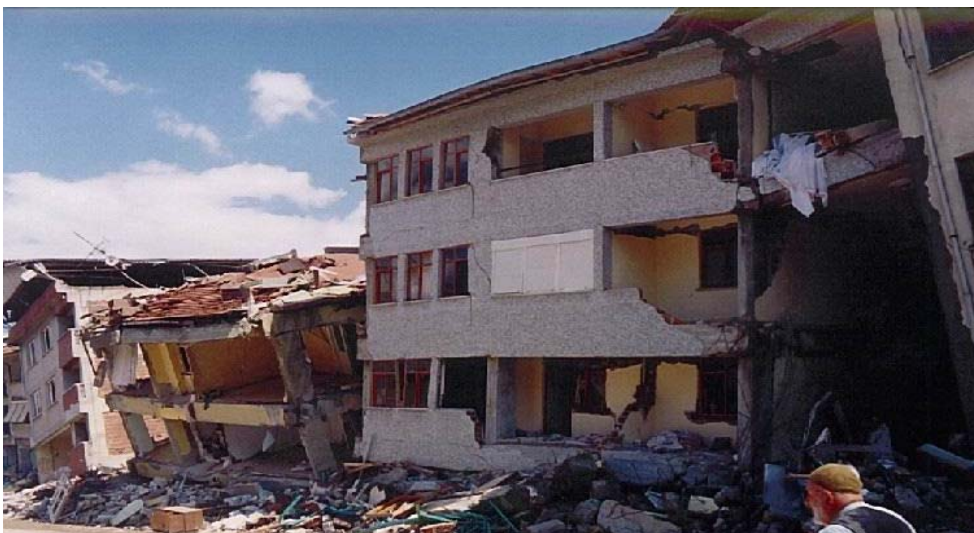
Figure 4: Semi-collapsed buildings in Adapazari, which were to be demolished soon [iii].
