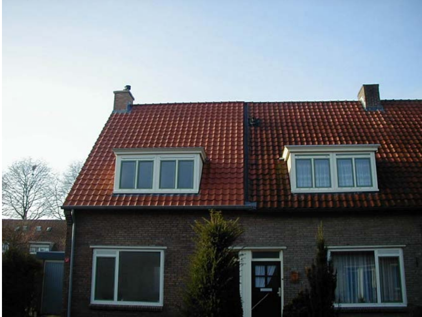
Figure 10 The project site, Lievendaal, after renovation (left) and before renovation (right)
