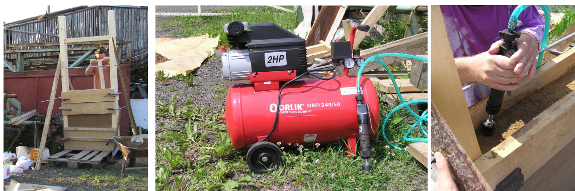
Fig. 6 Hand ramming with wooden rammer and technological equipment for machine ramming
