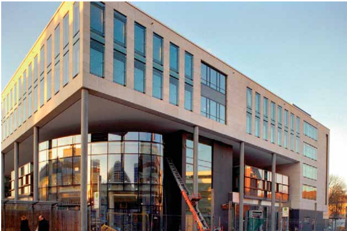
1 New building Sparkasse Hagen
