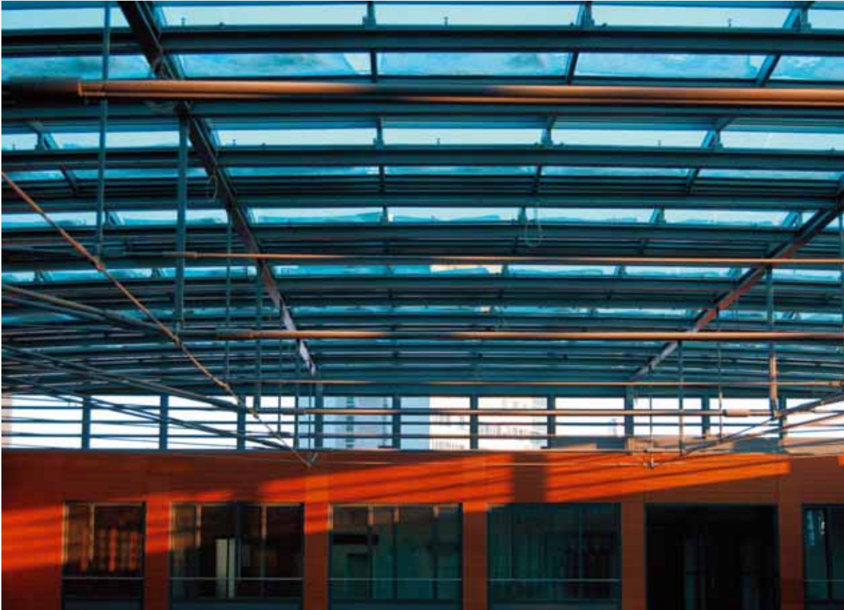
12 Roof structure with ventilation panels
