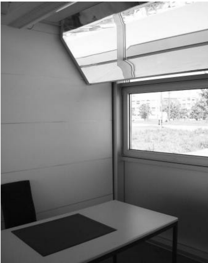
Figure 8. External and internal views of the integrated anidolic system set up on a test module (reference module visible in the same figure).
