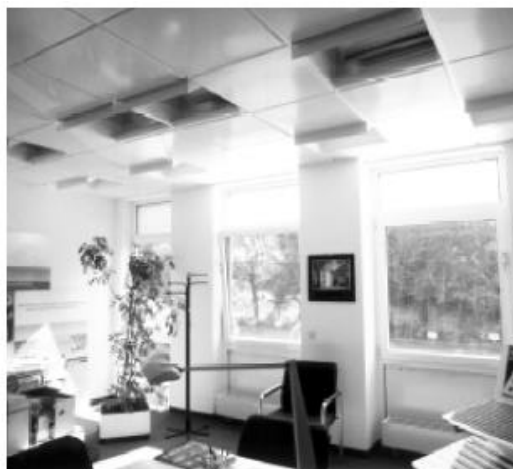
Figure 2. Sun directing glass attached above a normal viewing window (ADO office building Germany) (IEA 2000)
