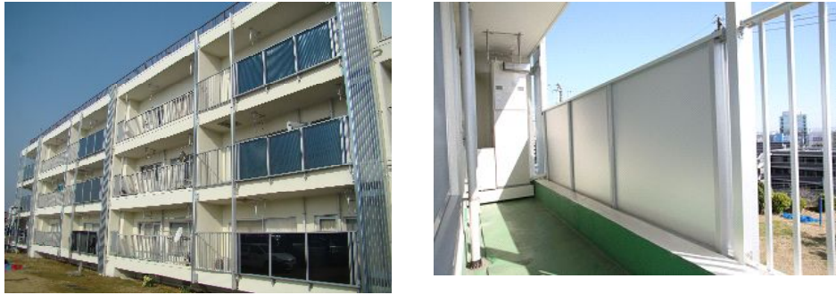
Fig.7 Appearance of solar thermal collectors installed vertically on balconies in test subject apartment-house
