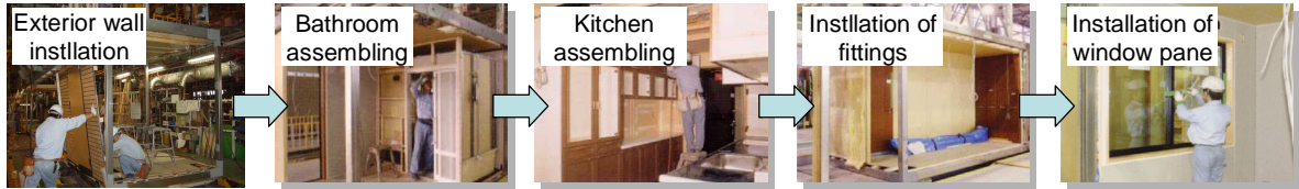
Fig. 3 Factory assembling of Heim Units
