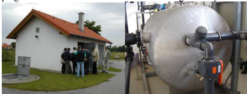
Figure 5 – Pumping station in Slovenia
