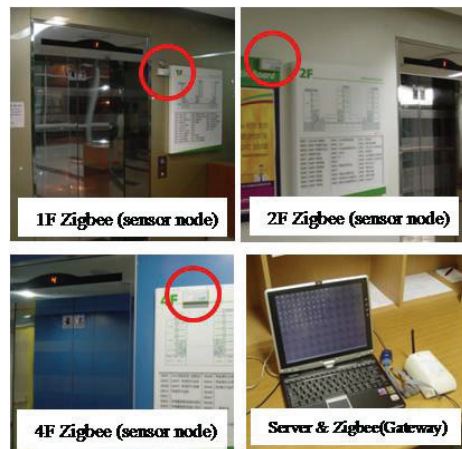
Figure 4 Installation of Equipment
