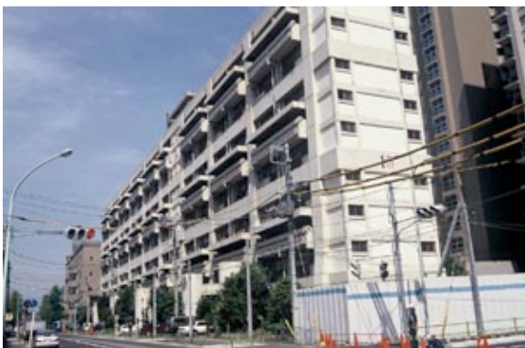
Figure 1 Harumi Apartment Building
