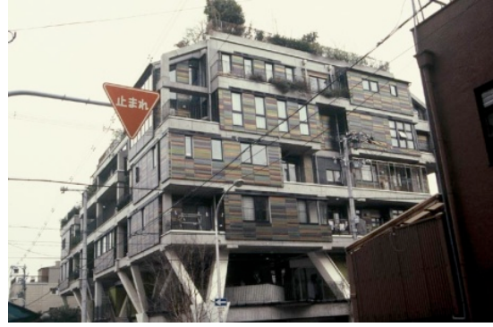
Figure 24 NEX21 after remodeling
