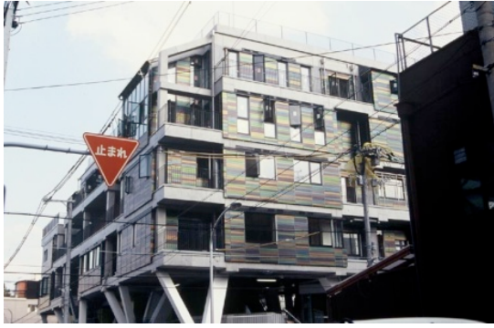
Figure 23 NEX21 before remodeling
