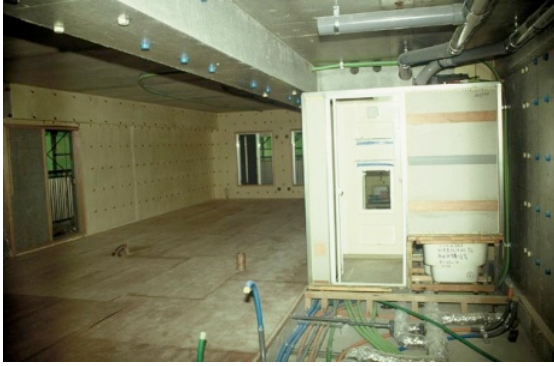
Figure 15 CHS Teradamachi Apartment
